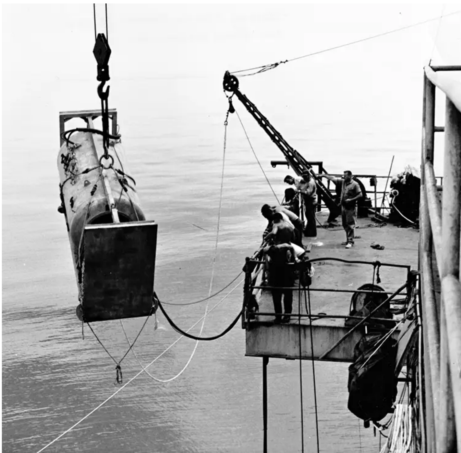
Lowering the Personnel Transfer capsule (PTC) to Sealab I.
